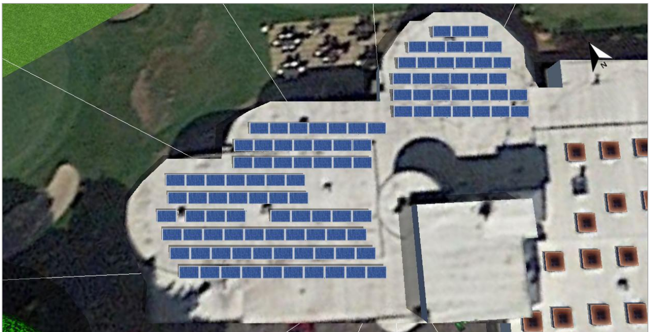
Figure: 1. Module Area - Arbitrary Building 01-Mounting Surface Southwest
